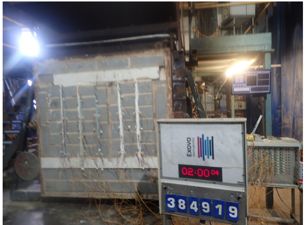
The unexposed face of the wall construction after a test duration of 120 minutes
