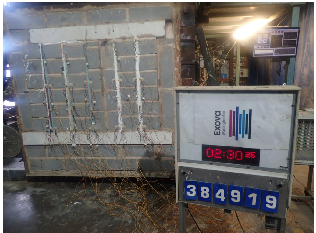
The unexposed face of the wall construction after a test duration of 150 minutes
