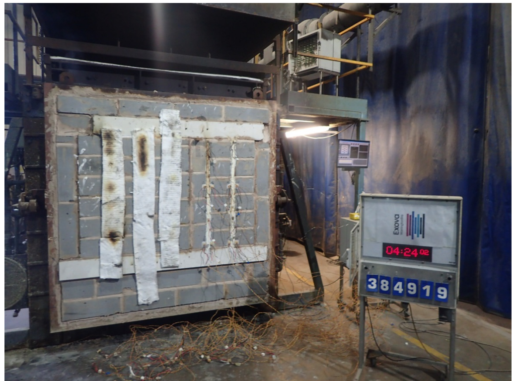
The unexposed face of the wall construction after a test duration of 264 minutes
