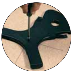
Setting-up The diameter of the finished access hole will be 250mm. Carefully mark the centre point of the circle, if possible positioning the access hatch between the floor joists. Screw the Routabout jig to the floor using a single No.8 particle board screw at the centre point to act as a pivot.
